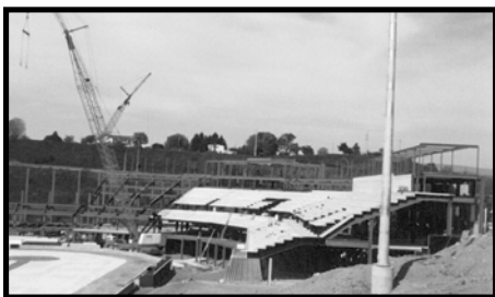
Blair County Ballpark under construction, Fall 1998
